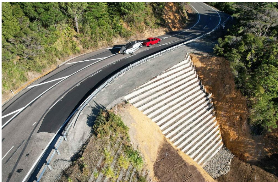
Recently stabilised underslip at Pumpkin Hill near Tairua
